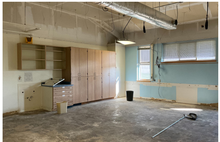
Demolished ceilings and floors make way for renovated classrooms.
